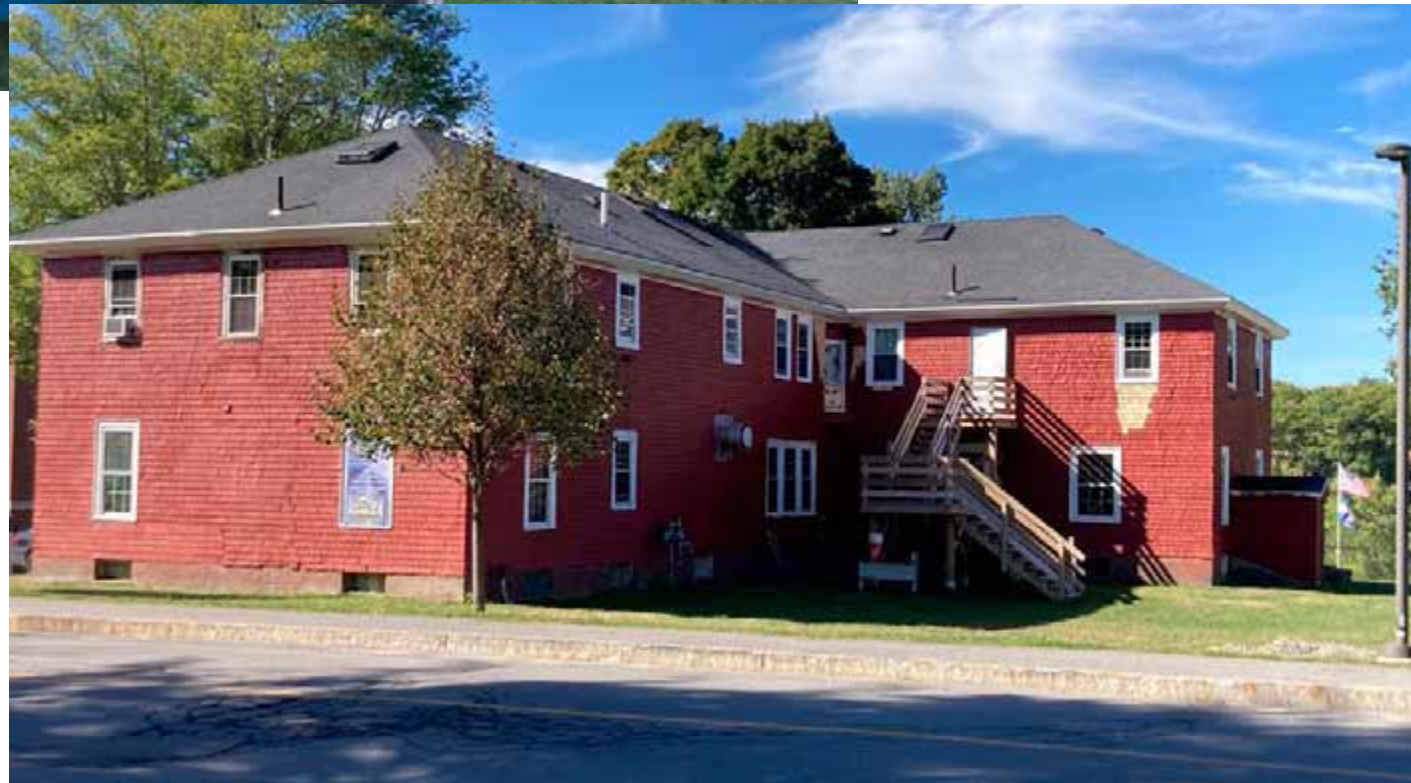
922_NEW_ViewFromWells_2891.JPG — (Small areas have been done since photo.)
