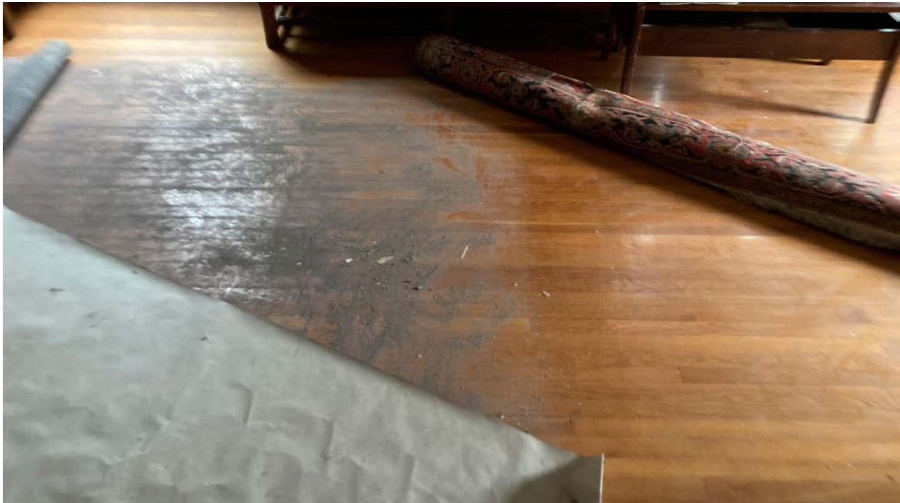
At left, mostly fine dust from deteriorating rug pad. At right, pad was discarded and floor cleaned in July of 2021 and appears here as I left it then.
