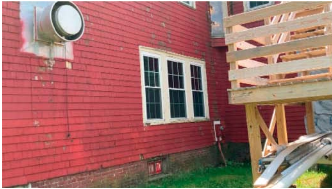
617-4 KITCHEN WALL 2441.MOV
